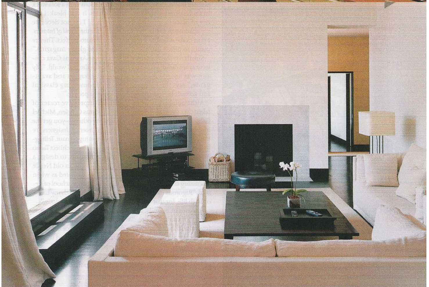
Central Park West Apartment: Living Room Fireplace. In Spring 1999 our Principal Restored Several Fireplaces and Chimneys for Giorgio Armani.
